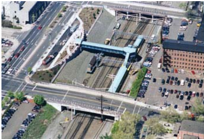
Aerial view of new commuter rail station at State Street, a component of the New Haven Harbor Crossing intermodal project.
