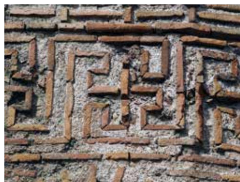
Fig. 5 Swastika ornament executed in brick, South church of Constantine Lips monastery, photo: J. S. Ćirić
