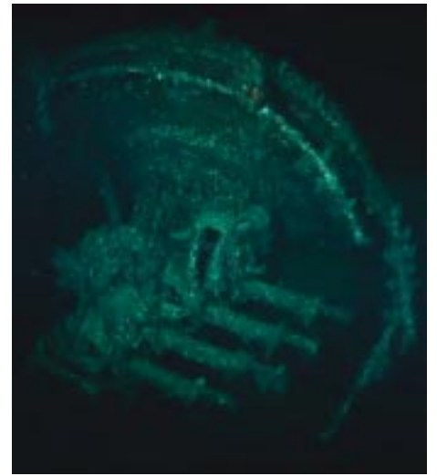
Anti-aircraft guns protected the bridge area
