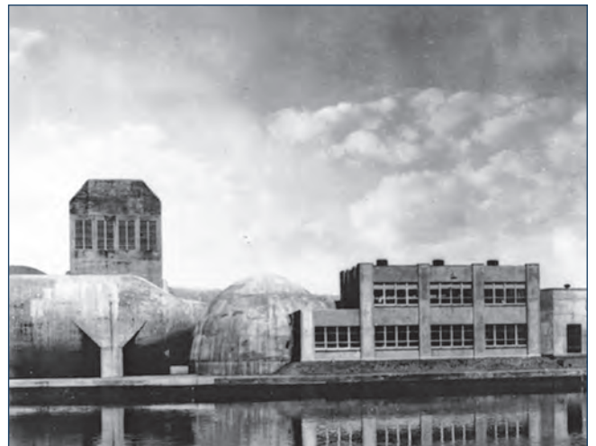
The 8-Foot HST at the NACA Langley Aeronautical Laboratory provided the means for testing large models and some full-scale components at a simulated speed of 500 miles per hour. (Image Number GPN-2000-001821)
