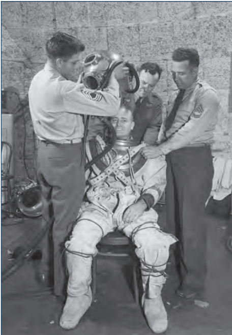
NACA physicist Ray Wright suits up in a deep-sea diving suit in preparation for entering the test section of the 8-Foot HST. (Image Number NASA L-64110)
